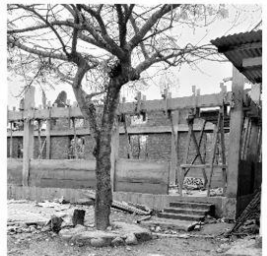
Julia's Memorial Chapel under construction
